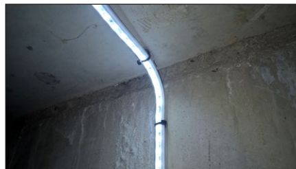
quickly fastened by means of plug-in dowels in the shaft head flexibly around the corner
